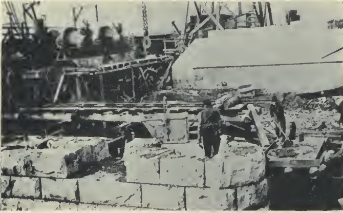
Fig. 2.—Pier B and north abutment.
